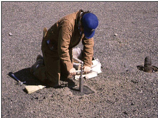
Coring a roof to verify infrared findings.
