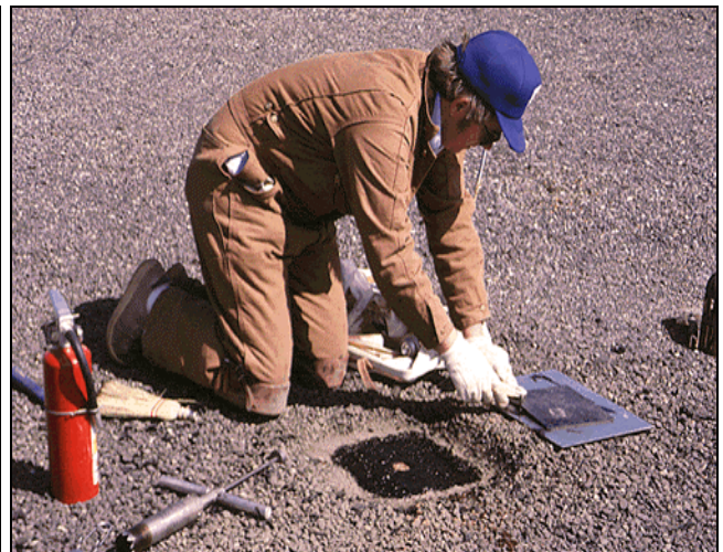
Patching a roof after coring.
